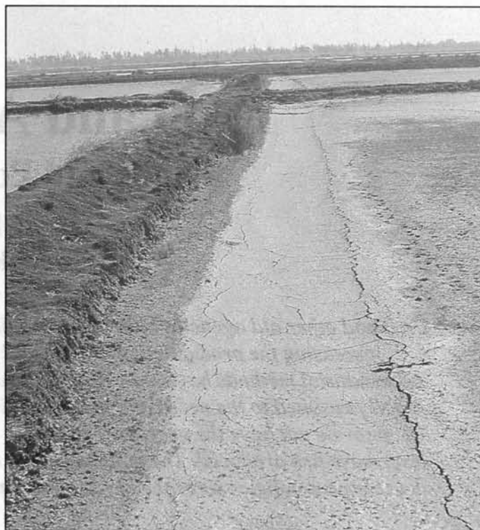
View along the bank of one of the production ponds at the FAO El Zawiyah Demonstration Fish Farm, Egypt. This shows the extreme erosion of this bank, which was only in use for a few weeks before the photograph was taken. The bank originally had a 1 in 3 slope from its top to the extreme left edge of the picture; the slope is now less than 1 in 20 where it had been covered in water. (Photo: D. Cross)
