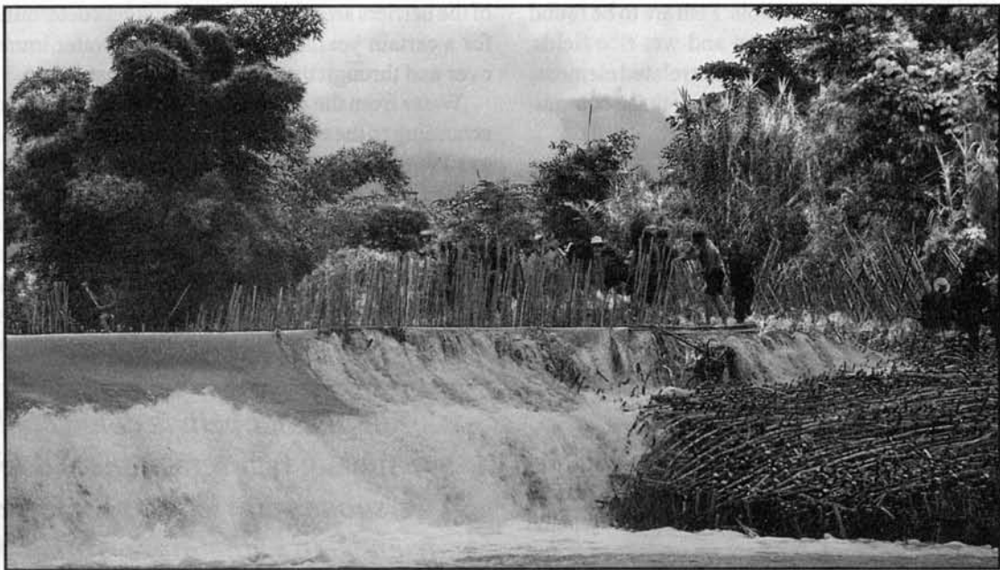
Villagers build a traditional wooden water-barrier to hold back water in a muang faai reservoir. Muang faai water-management systems enable villagers to divert, store and divide swift streams so that they can be used in wet-rice agriculture. A study of these systems shows the many complex interrelationships between communities, technology, production and natural resources. (Photo: Chatchawan Tongdeelert)
