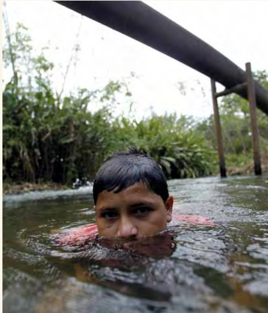
A young boy swims under an oil pipeline in Ecuador
